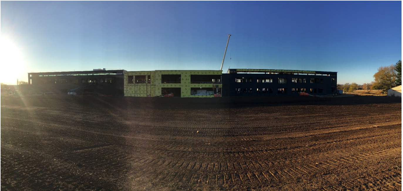
Flex Café Sheathing is wrapping up and Glazing installation is beginning on Area A.
