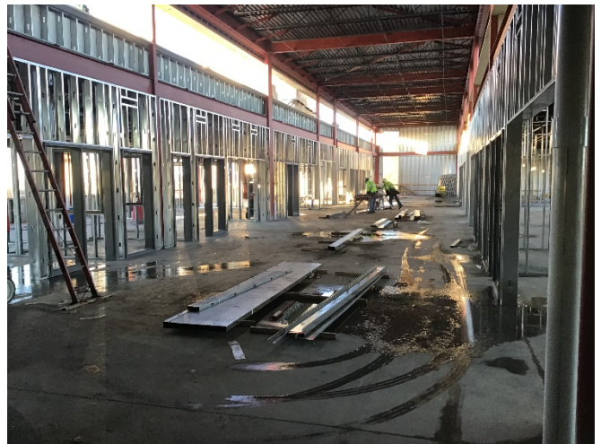
Interior Wall framing on Level 2 of Area A.
