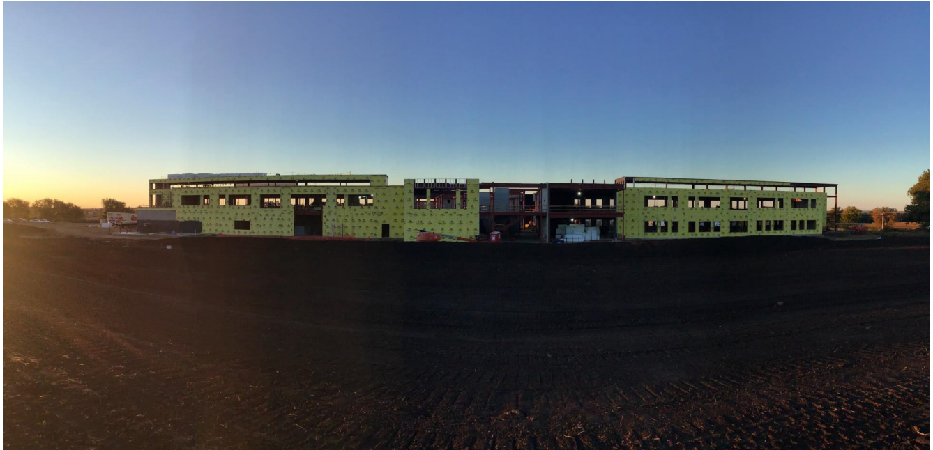
AVB installation is making its way around Area B. Exterior wall panels are up for Area A. Roofing has begun on Area B.
