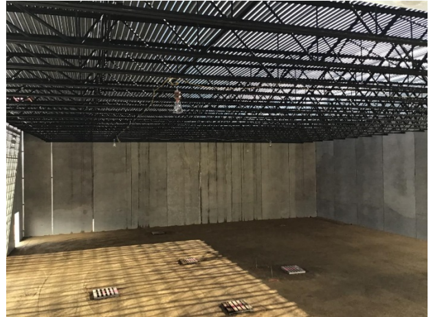
Gym Joists, Decking, and Grading.
