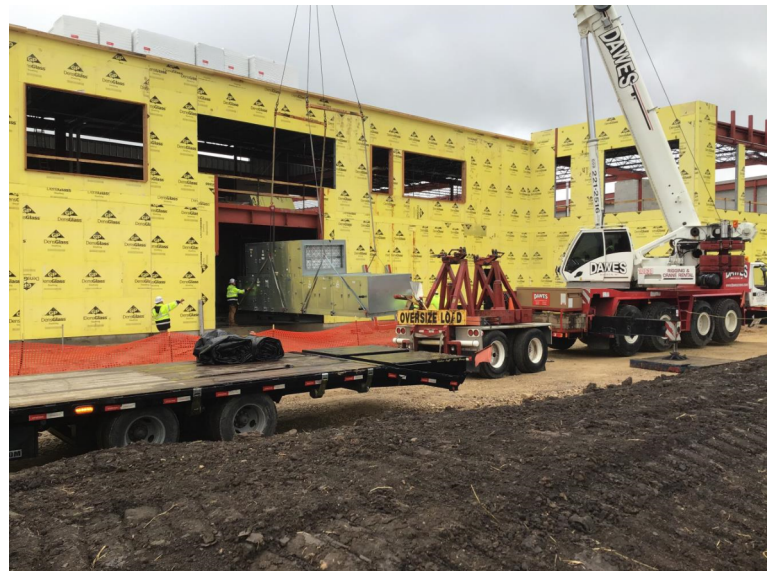
Mechanical Unit being set in the mechanical room.
