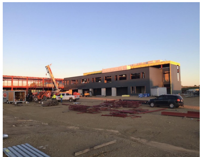
AVB Sprayed on the South and East sides of Area B.
