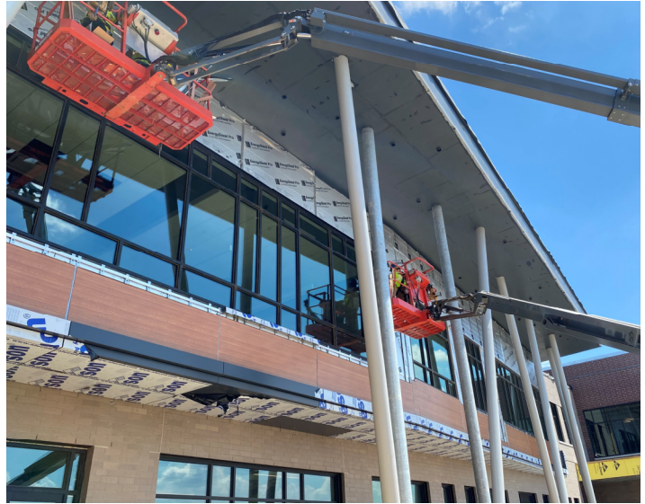
Installation of Exterior Metal Paneling
