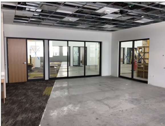
Classroom sliding glass doors are in progress of being installed.
