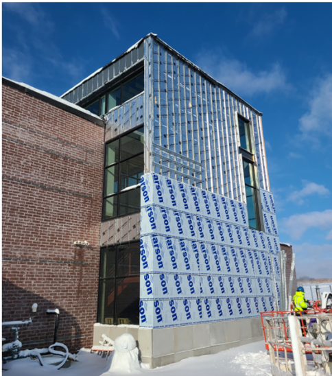
B Stairwell Metal Panel Install
